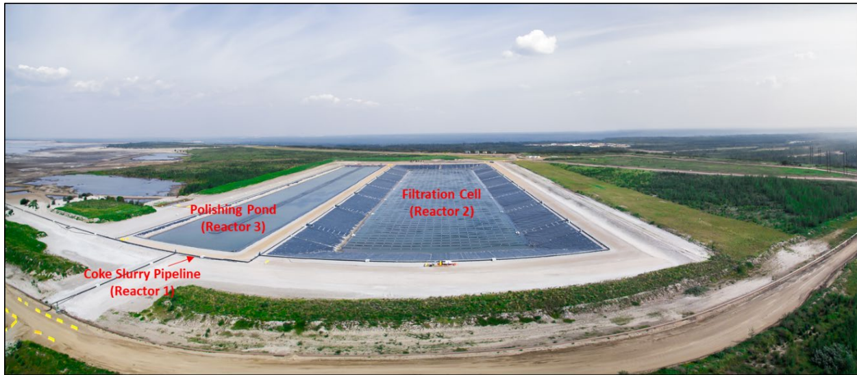
Figure 3: Treatment facility for the 2019 Water Return Demonstration Project.
